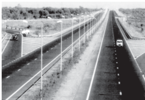
Fig.7.2: Ahmedabad- Vadodara Expressway
