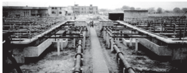
Fig. 6.11: Sewage Treatment plant under Yamuna action plan at Faridabad
